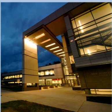
Night, exterior canopy lighting
